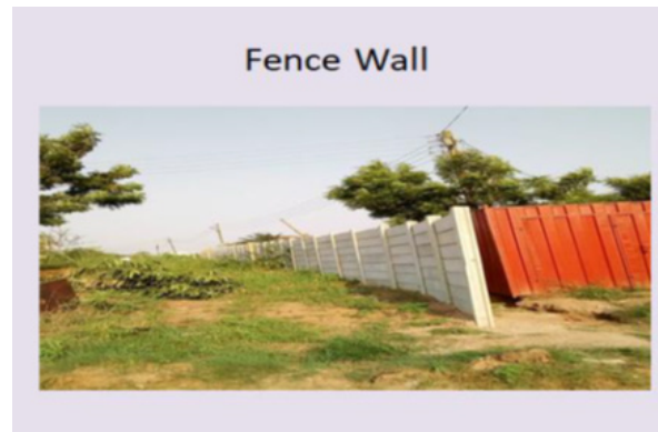
Fencing of the Hospital
