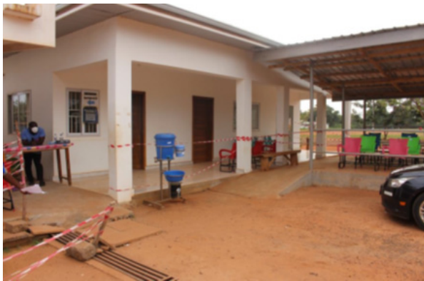
Construction of new pharmacy block
